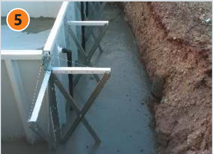
Pouring concrete onto panel supports appropriate for the pool project.
