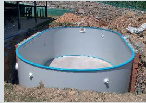
3 Assembly of the steel body in accordance with the pool project.
