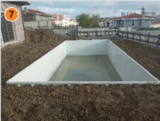
Filling the pool area in accordance with the pool project
