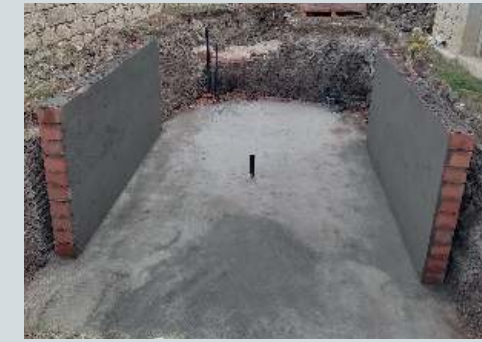
2 Pouring infrastructure ground concrete and construction of side walls
