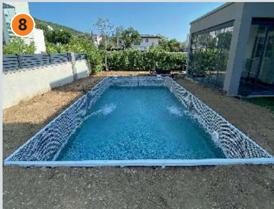
Covering the pool with antibacterial PVC Liner
