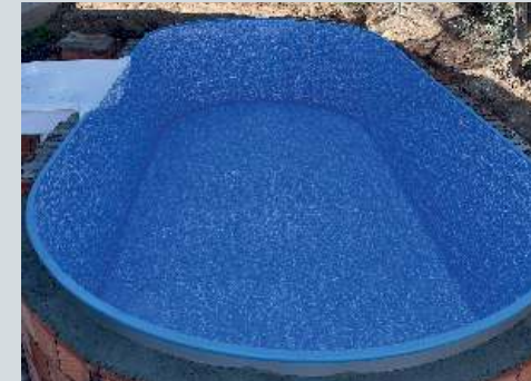
4 Covering the pool with a single piece antibacterial PVC liner
