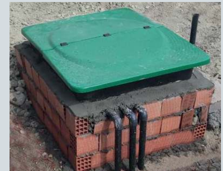
6 Preparing the location of the engine room and protecting its surroundings
