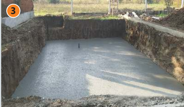
Pouring infrastructure ground concrete suitable for the pool project
