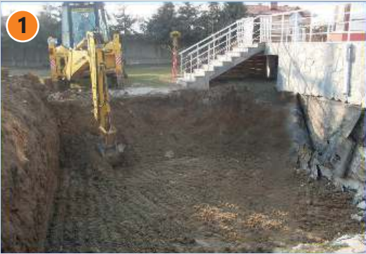
Removal and disposal of excavation material suitable for the pool project
